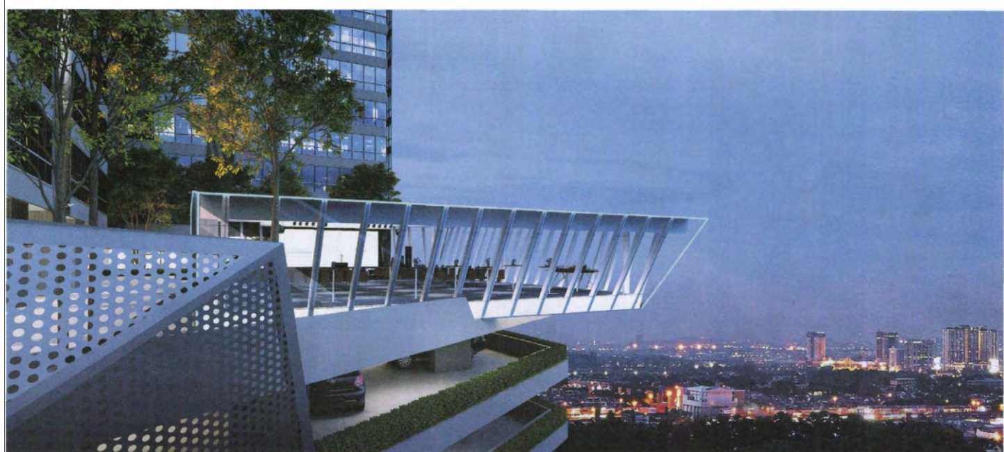
The upcoming MET Corporate Towers within the KL Metropolis will consist of premium grade office spaces – in terms of amenities and design – and will cater to discerning tenants and businesses
